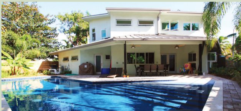
Moreland on Trapp, which features doors and windows by CGI, is the first LEED Platinum single-family home in the city of Miami.
